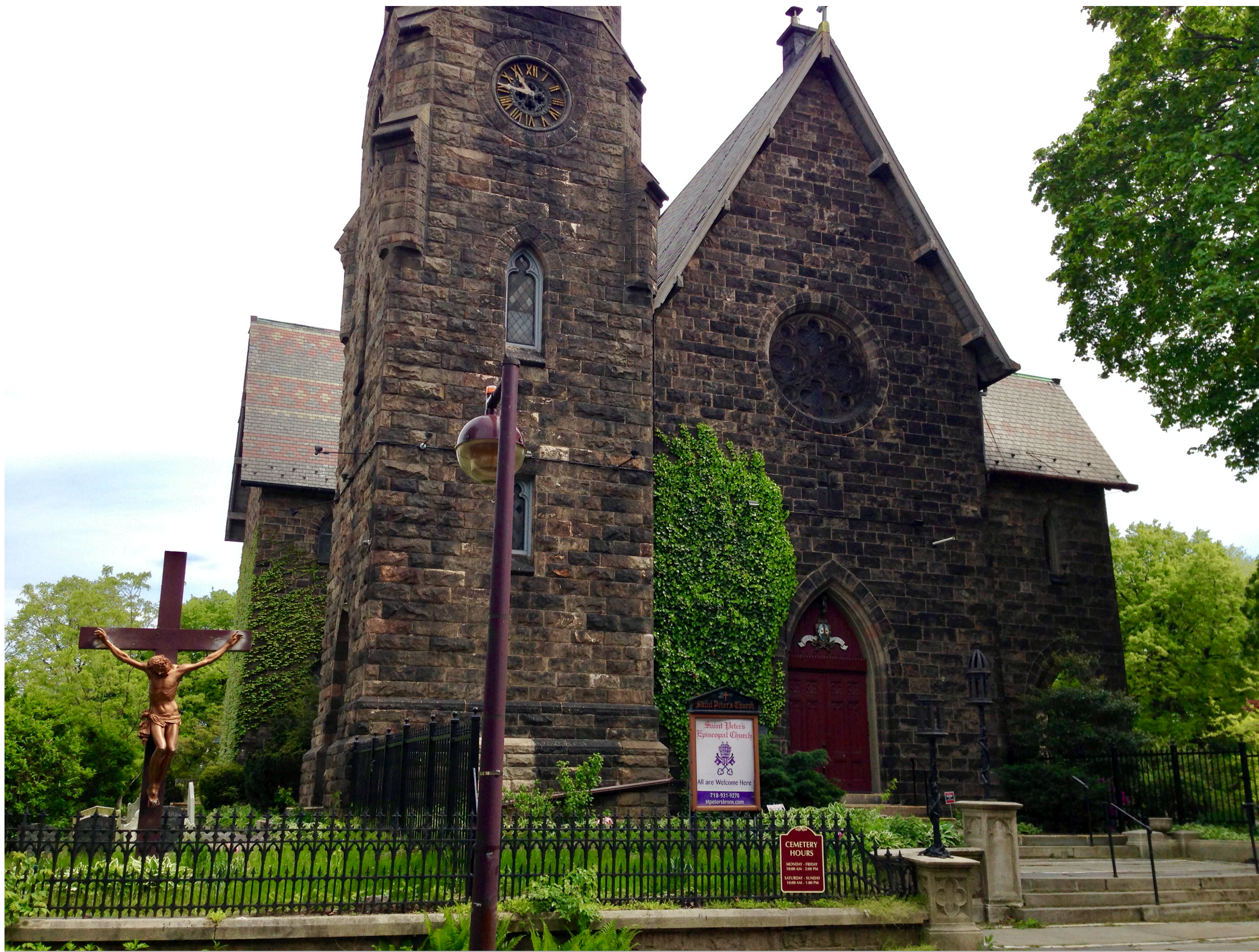
Saint Peter's Church, Chapel, and Cemetery Complex, Westchester Square, Bronx, N. Y., circa 2017. Photograph by Hugo L. Gonzalez
