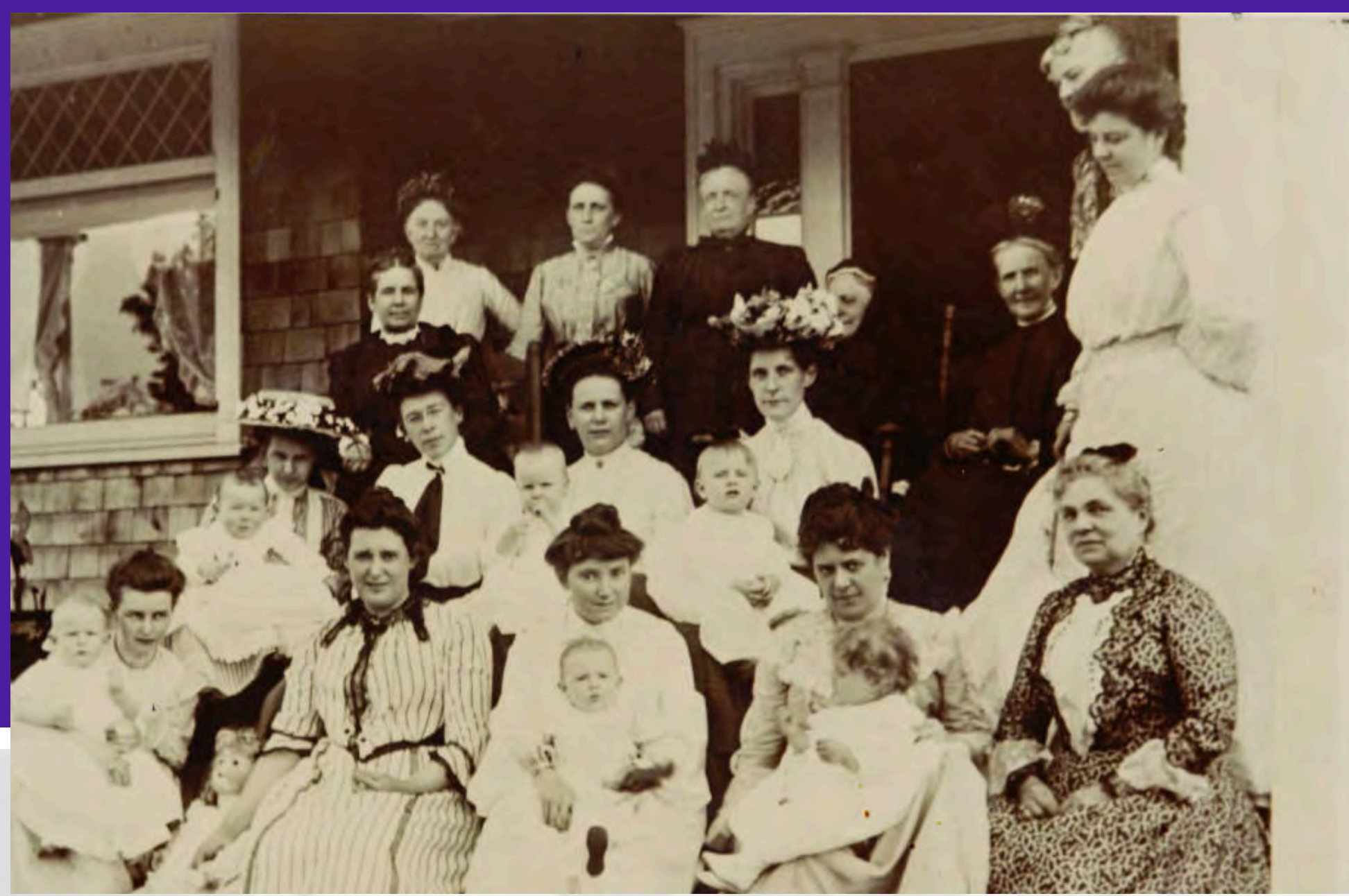
34 Drake Road where the women sit on the steps (right). The demolished property became the field at Drake-Edgewood park.
