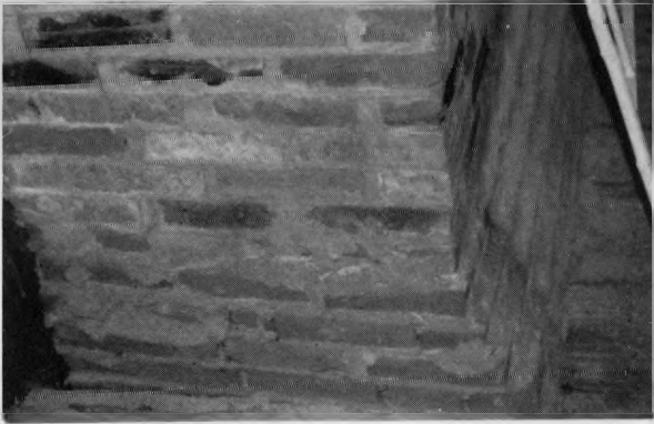
Southeast Chimney Base in Attic
