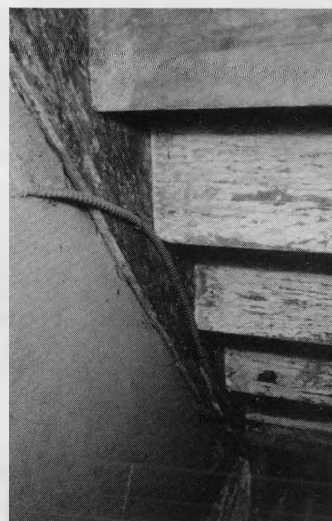
The old door opens to the cellar stairway.
